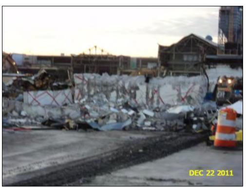
A-12: Demolition view - Looking southeast at B-Bank during Building 2 demolition. The PCB-impacted concrete (marked with the red X's) was segregated from other demolition debris.
