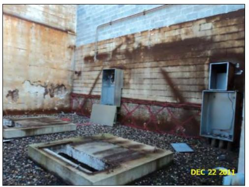
A-17: Looking northeast at the east wall inside C-Bank. The PCB-impacted concrete (marked with red X's) was segregated for proper disposal.
