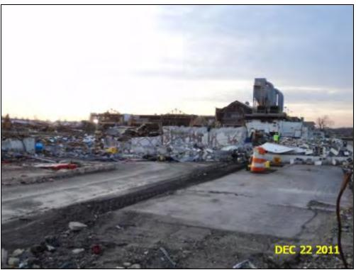
A-13: Demolition view - Looking southeast at B-Bank during Building 2 demolition. The PCB-impacted concrete (marked with the red X's) was segregated from other demolition debris.
