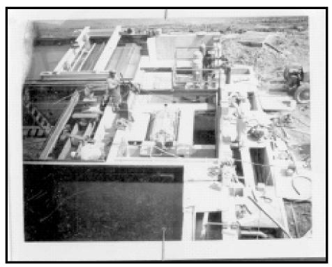
**Photo 21** – Undated photo. View looking north from WWTP roof at new Microscreen installation. Pipe trench is present along east side of tanks and is partially covered and north settling basin is full.
