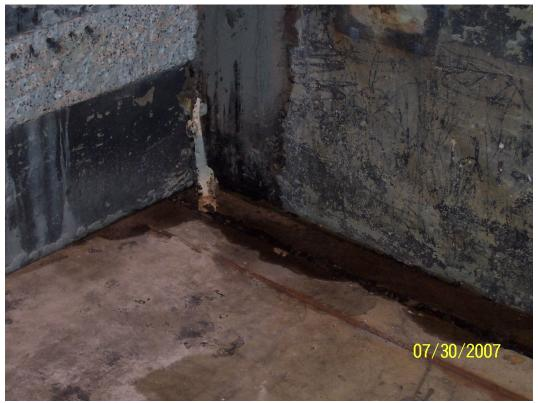
Photo 4 – Possible crack in the southeast corner of basin, where a boring was later placed in the floor.
