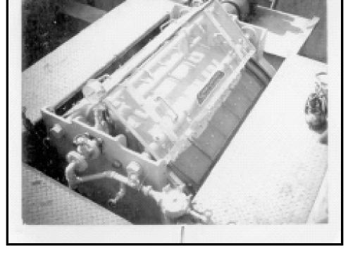
**Photo 19** – May 8, 1972 photo. View looking northwest from WWTP roof at new Micro screen and effluent discharge point (northeast corner of Oxidation tank). Pipe trench is present on the right-hand side.
