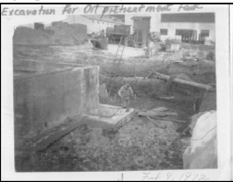
**Photo 6** - February 9, 1972 photo. View looking northeast from near north mandoor of WWTP building. Note former sump pad and excavation for new EQ tank.
