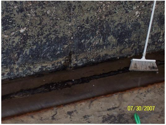
Photo 5 – Possible crack in wall along the south side of the basin, where another boring was placed.
