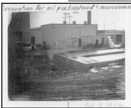
**Photo 3** – February 9, 1972 photo. View looking Southwest toward north side of Bldg 41. Excavation for new EQ tank is shown in the foreground. Note that the two new settling basins have already been constructed and are filled with water.
