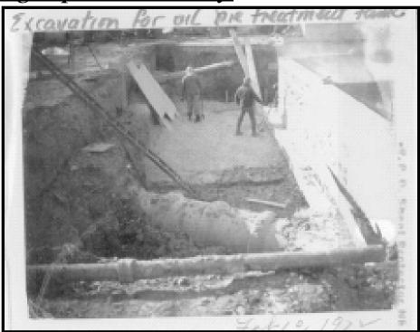
**Photo 8** - February 1972 photo. View looking south from northeast corner of new Settling tanks. Note 30" diameter underground stormwater pipe and smaller sanitary pipe. Workers are standing on new base for pH adjustment tank.
