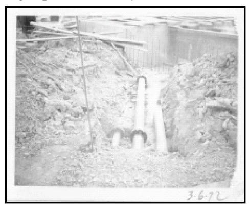
**Photo 12 -** March 6, 1972 photo. View looking southwest toward the northeast corner of the EQ tank. The three pipes are presumed to be from Bldg 2 WW tank area. Rebar from Neutralization tank wall construction in background.
