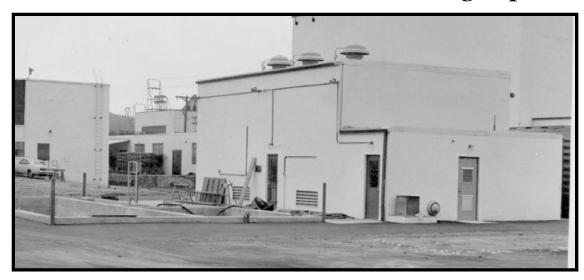
Photo 1 – Undated, believed to be the originally constructed Building 41 WWTP and open tanks circa early 1969 (following construction); view is looking southeast. Features in Photo 1 are consistent with 12-5-67 AMF Dwg 61-7-60000 (Figure 1). Note only one settling basin is visible and adjacent to a smaller treatment tank (both empty and all concrete, in-ground, open topped tanks).
