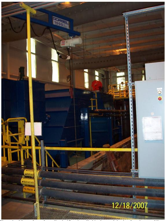
Photo 9 – View of new Lamella clarifiers installed in the north basin after closure. View facing northeast.
