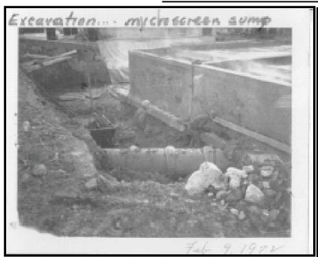
**Photo 5** – February 9, 1972 photo. View looking southwest along east side of new settling basins. Note large 30" diameter stormwater pipe in foreground.
