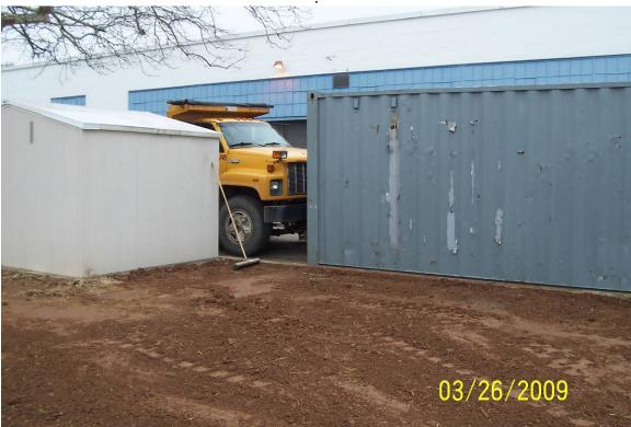
Photo 14 – Final closure of the vault. Compacted gravel overlain by topsoil, ready for seed by H-D trades.
