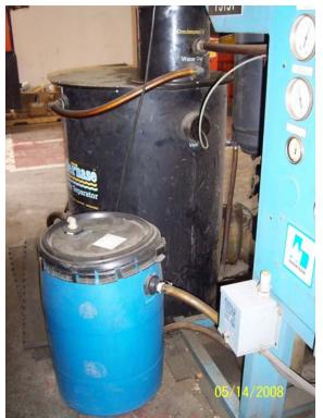
Photo 5 - Condensate knockout tank that was the source of water draining into the vault following cleaning. This water was redirected with a hose to discharge into floor drain in men's bathroom during the closure of the vault.
