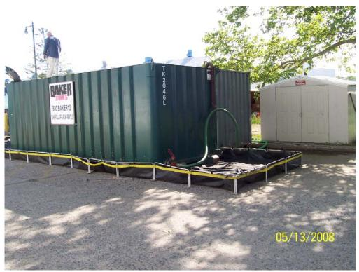
Photo 4 - Liquids from Building 45 vault pumped into Baker Tank located next to vault.
