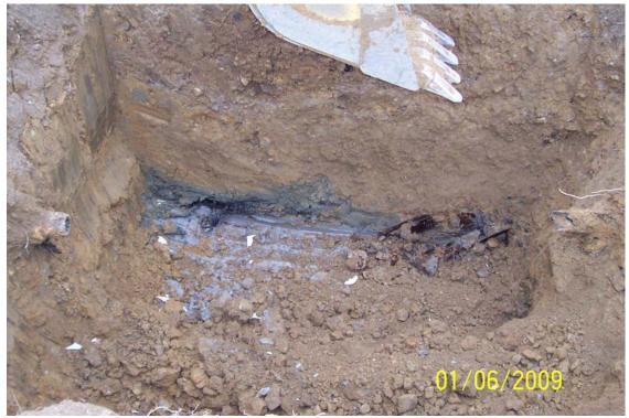
Photo 11 - East wall of excavation-stained and/or gleyed soil and wood debris visible.
