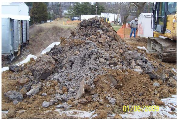
Photo 12 - Excavated gleyed/stained soil from east wall of vault.
