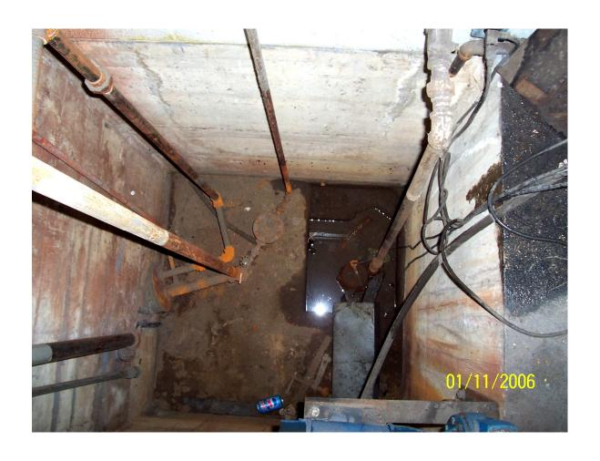
Photograph 2 – Concrete pit and sump pump in the southeast corner of Building 57.
