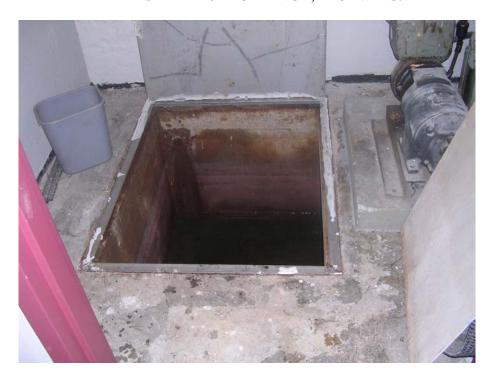
PHOTO 2 – VIEW OF SUMP B-16C LOOKING EAST, LOCATED WITHIN THE BASEMENT OF BUILDING 1, EAST WING. THE WATER ENTERING THE PIT IS CONDENSATE FROM SUMP B-14.
