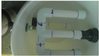
11. For the split ring hole, you will need to mark the center of the bottom bulkhead and just below the "W" screened piece.
